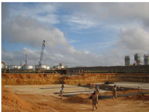
Acciona workers preparing the construction site
